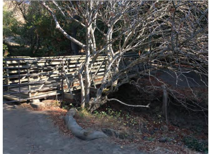
Description: Remove 5 wood pedestrian bridges. Replace 4 bridges that cross Dry Creek with new fiberglass bridges. Staff will replace the north bridge with a natural stone ford crossing a small tributary to Dry Creek.
