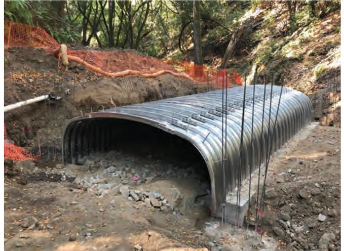
Description: Mitigation for environmental impacts under the Trails, Creeks and Ponds permit. A failing metal pipe culvert at Huckleberry Creek will be removed and a new creek crossing will be built with focus on enhanced storm water flow, sediment transport, fish passage, riparian habitat and creek bed resilience.
