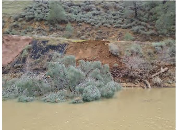
Description: Stabilize bank where a portion of the Dog Run Trail slid into the lake. Repairs will protect the trail and the utilities, including power to the raw water pumps, buried in the trail.
