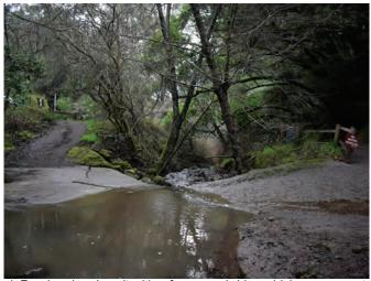
Description: Remove concrete crossing in Wildcat Creek at Brook Road and replace it with a free-span bridge which can support
