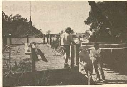
EBRPD Construction crew lowers Temescal pier into place.
