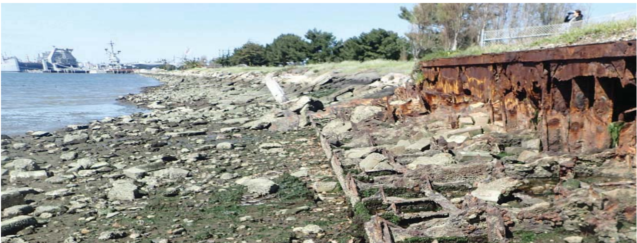
View 6: Rusted barge will be removed and slopes will be graded and stabilized.
