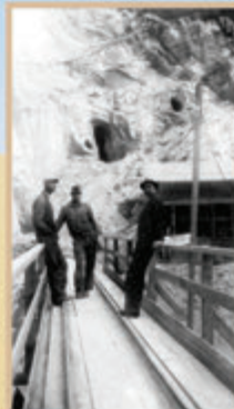
Left to right: Sand mill foreman Oscar Peterson, mine superintendent Albert Latham, and plant manager Joseph Bennett stand on the trestle structure at the upper workings.
