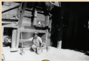
Sand mill operator Rex Peterson wears a respirator to protect himself from dust, a major hazard when working with silica sandstone, 1913.
