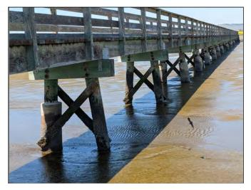
Repair damaged bridge timber piles with fiberglass jacketing and epoxy mortar. Repairing the two bridges will take place over several years to work within the tidal and environmental constraints. Description:
