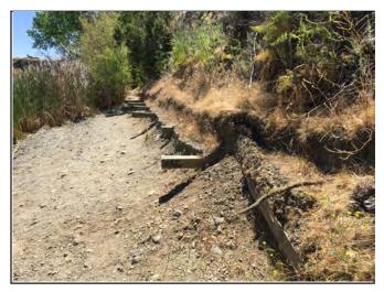
Description: Stabilize the slope under the lakeside trail that was damaged by heavy saturation of storm water.
