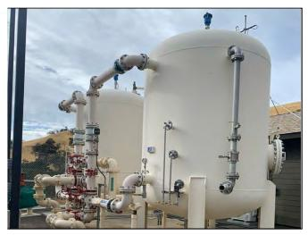
Description: Stabilizing the water system includes, repair the solids contact clarifier, replace several six inch control valves in the
