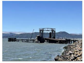
Description: Removal of the wooden Ferry Point Pier that has significantly deteriorated over several decades with many pilings
