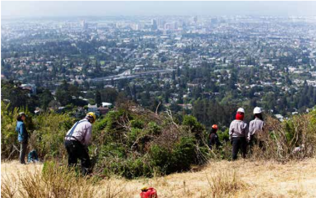
A crew clears brush as a preventative measure against potential wildfires.
