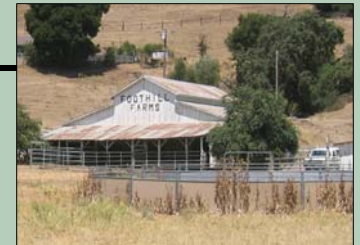
NEW - Tyler Ranch Staging area with picnic area, park residence & corps yard
