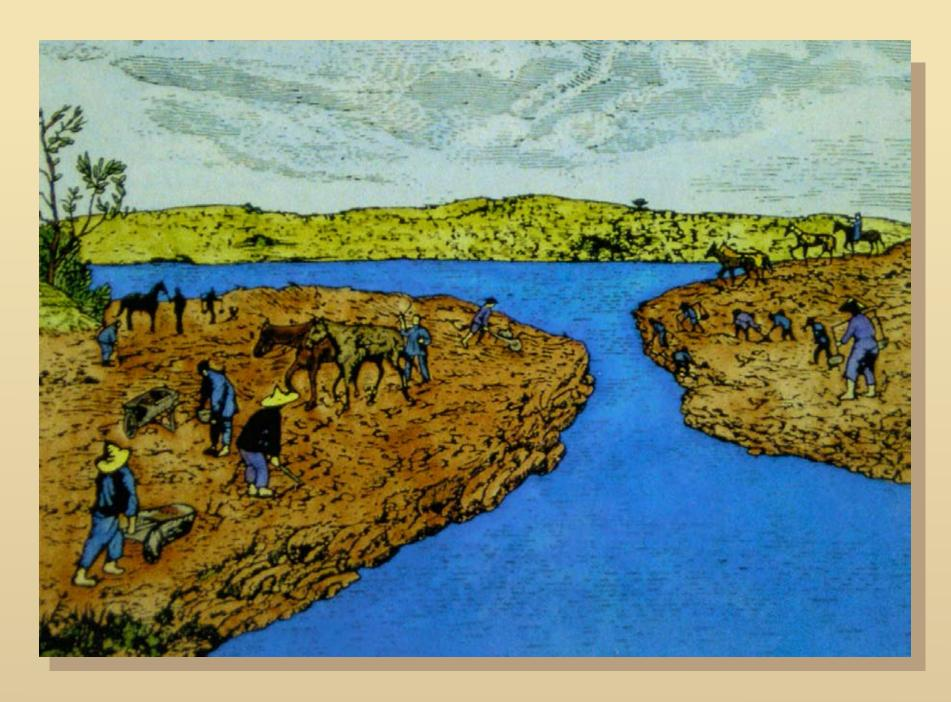
**Digging the dam:** To prevent leakage and the creeks' return, laborers dug three trenches, nesting one inside the other. The largest ditch was 900 feet by 150 feet; the second ditch or "puddlepit" was 90 feet from bank to bank and about 140 feet long creek-wise. In the third ditch, laborers constructed three concrete walls and then sealed the trench with concrete grout.
