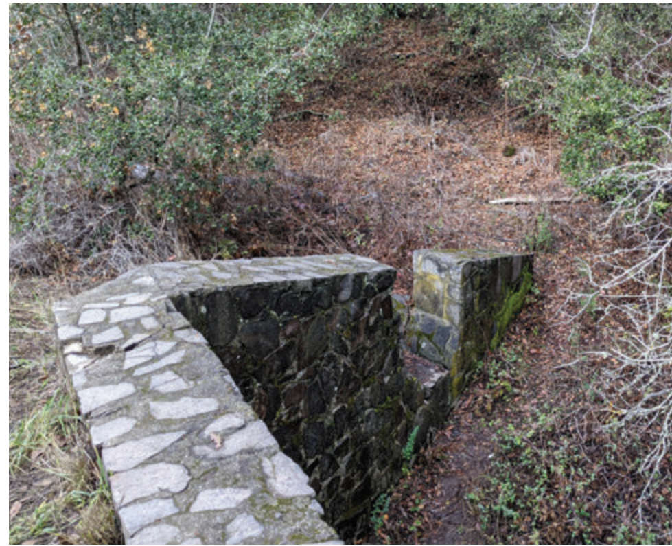
11 Jewel Creek WPA Headwall
