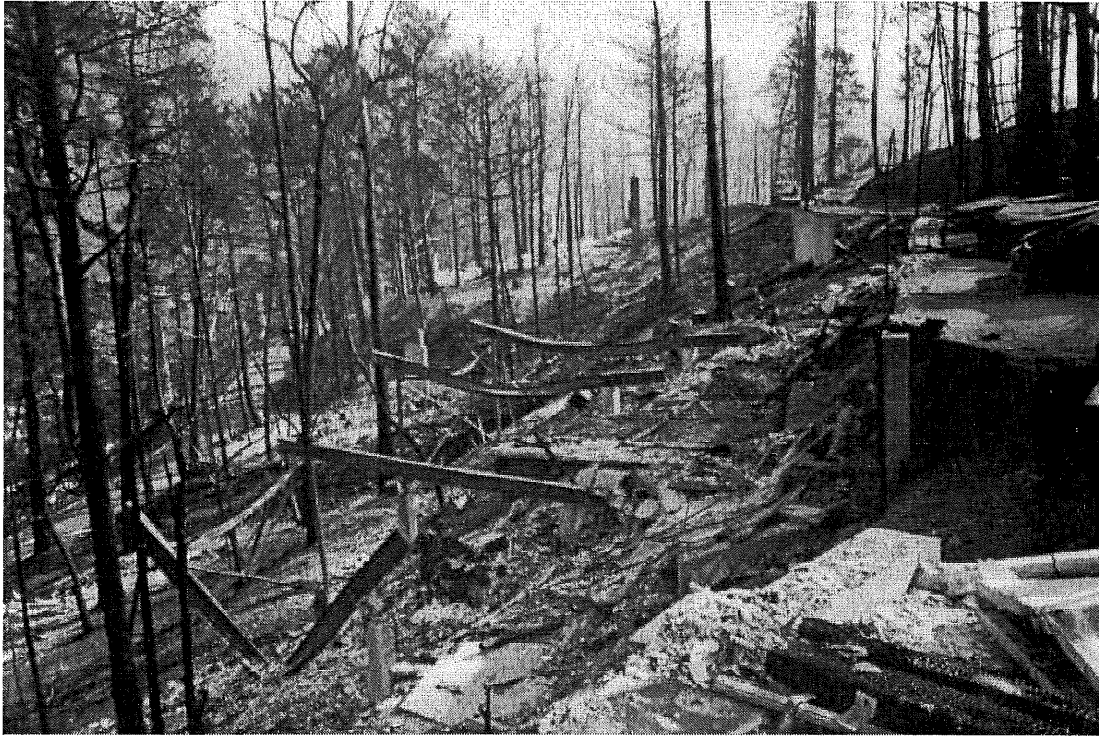
Buckled steel beams and burned trees, that appear to be seedlings from the 1970 fire, mark the location of a home on Buckingham Boulevard.
