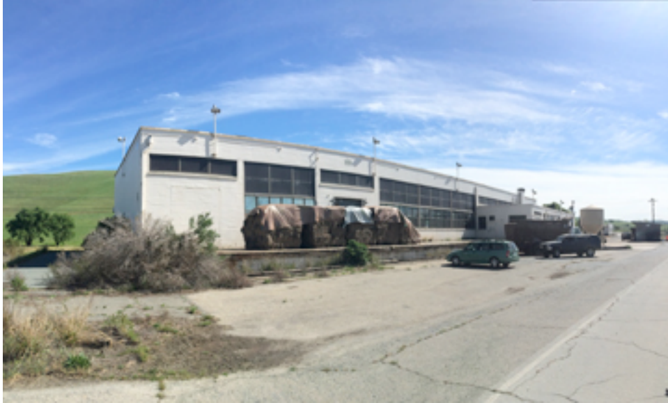
Building 1A-24: view of west façade
