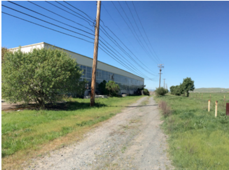
Building 1A-24: view of east façade from south
