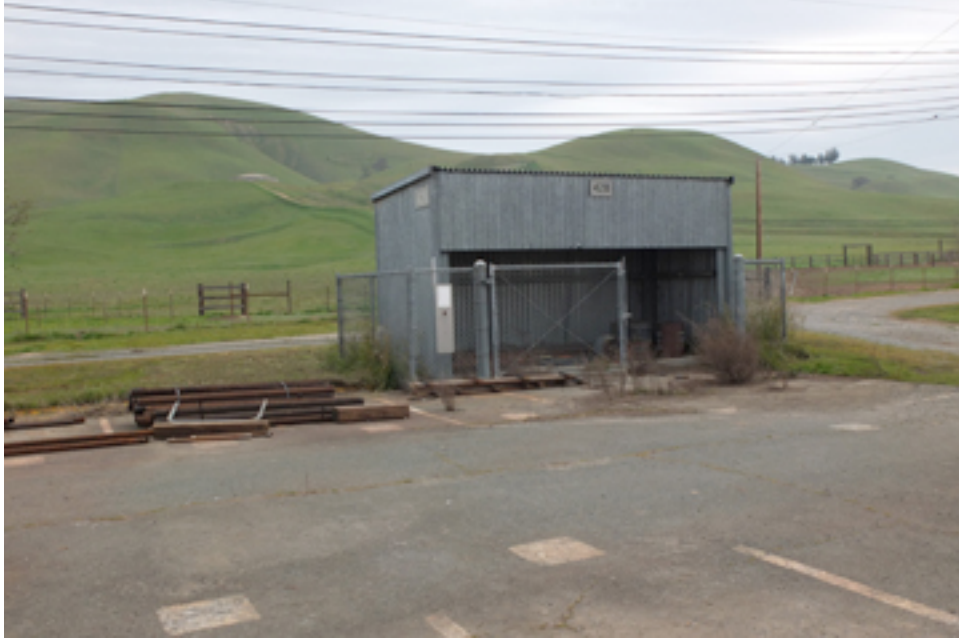
Building 428: view of west façade
