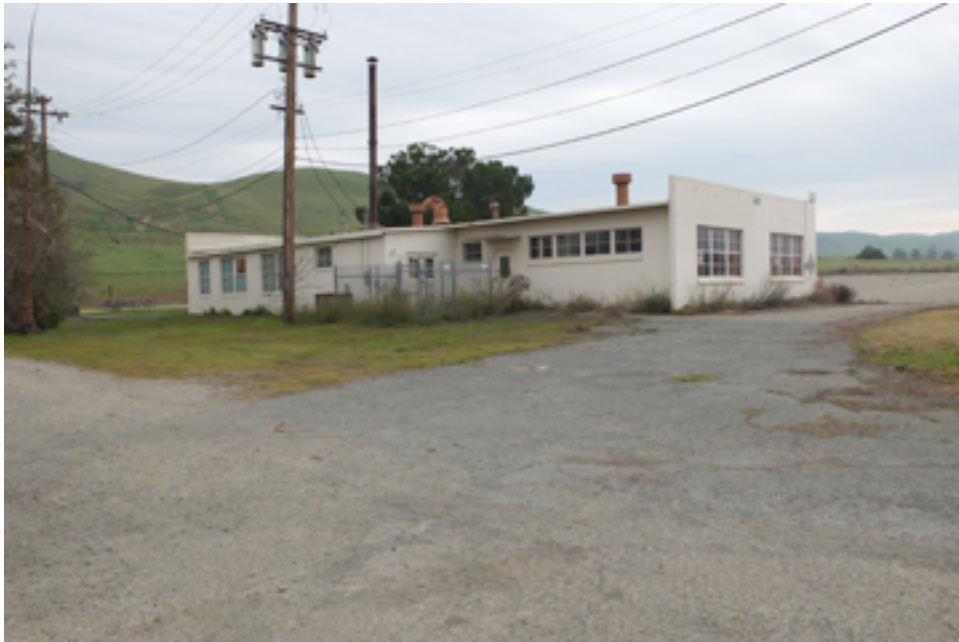
Building 1A-55: view of north and west façades
