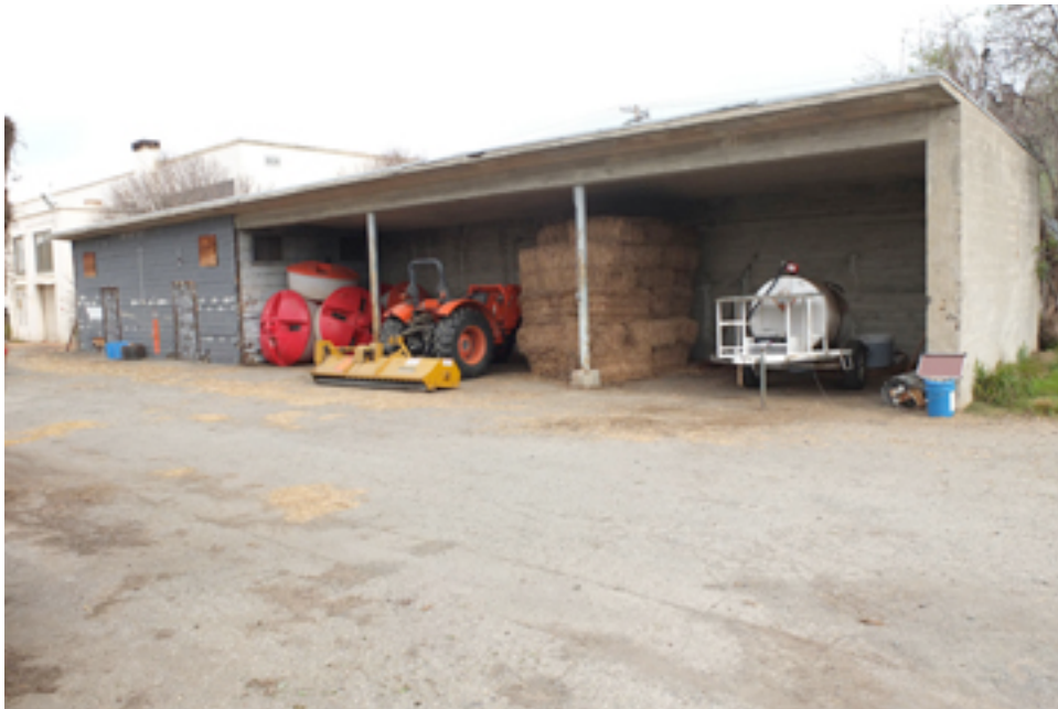
Building 1A-24B: view of west façade
