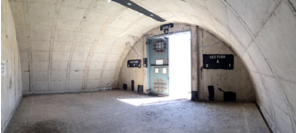
Typical Magazine: view of interior looking toward entry doors
