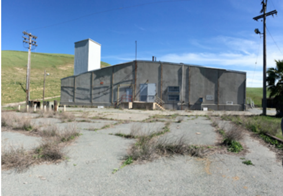
Building 87: view of west façade
