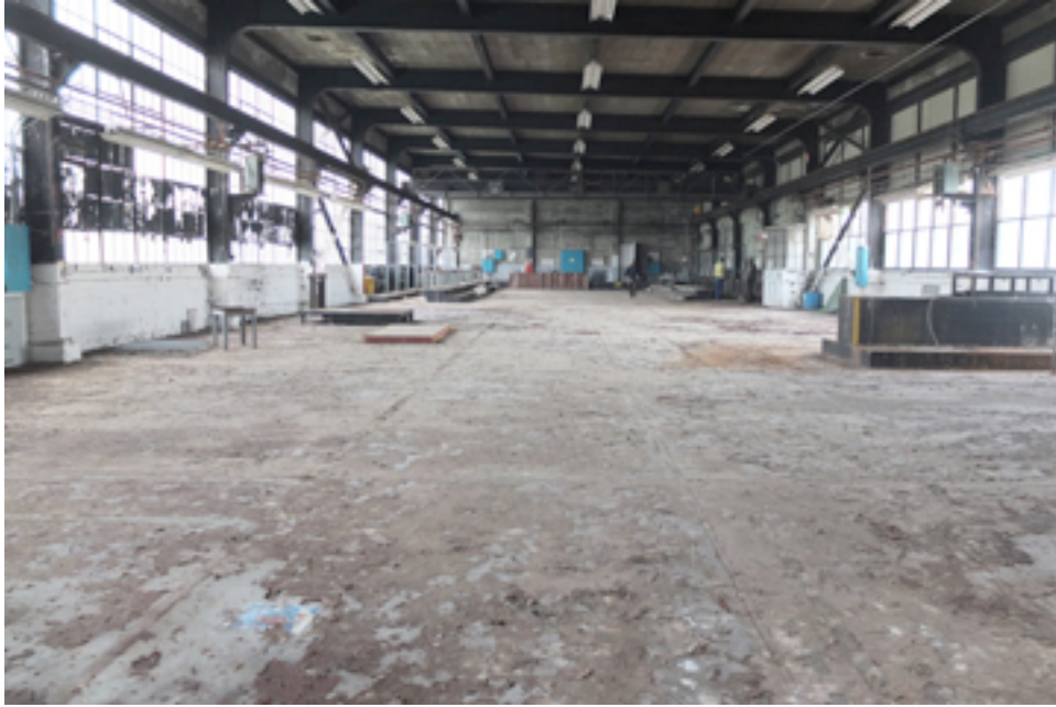
Building 1A-24: main interior space looking south
