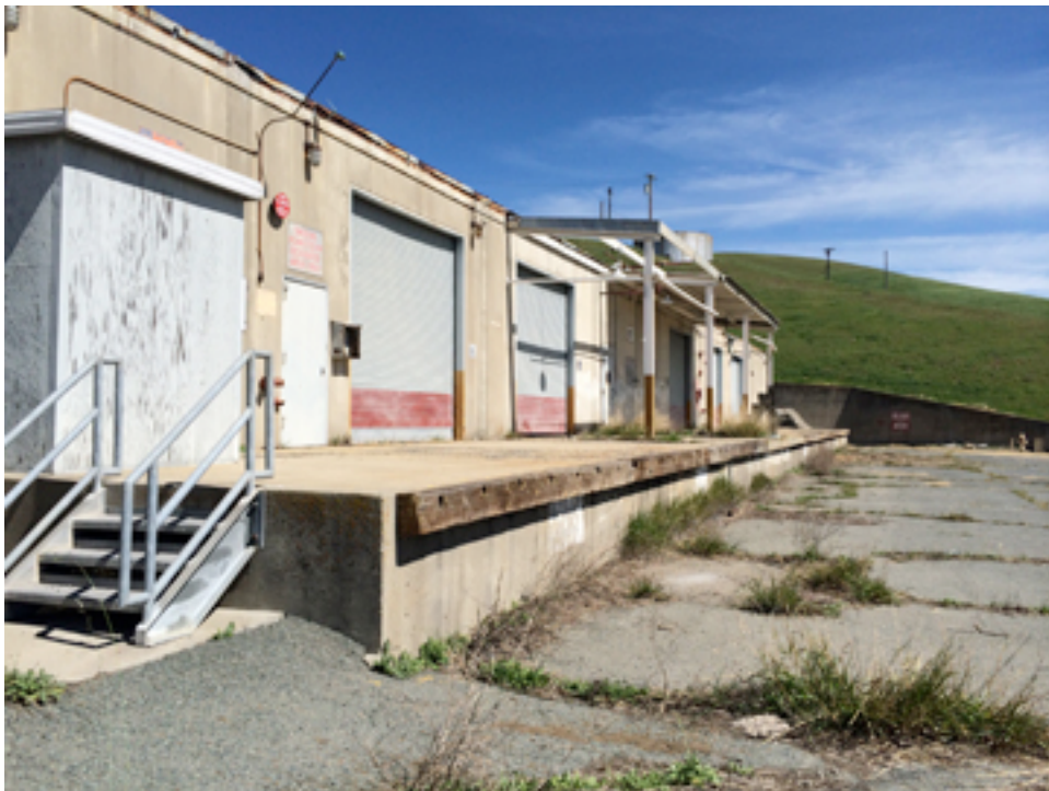
Building 87: view of south facade
