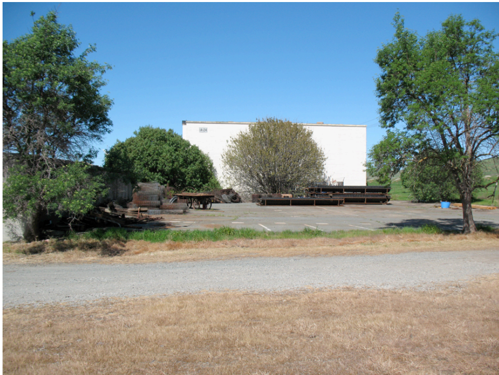
Building 1A-24: view of south façade and paved area
