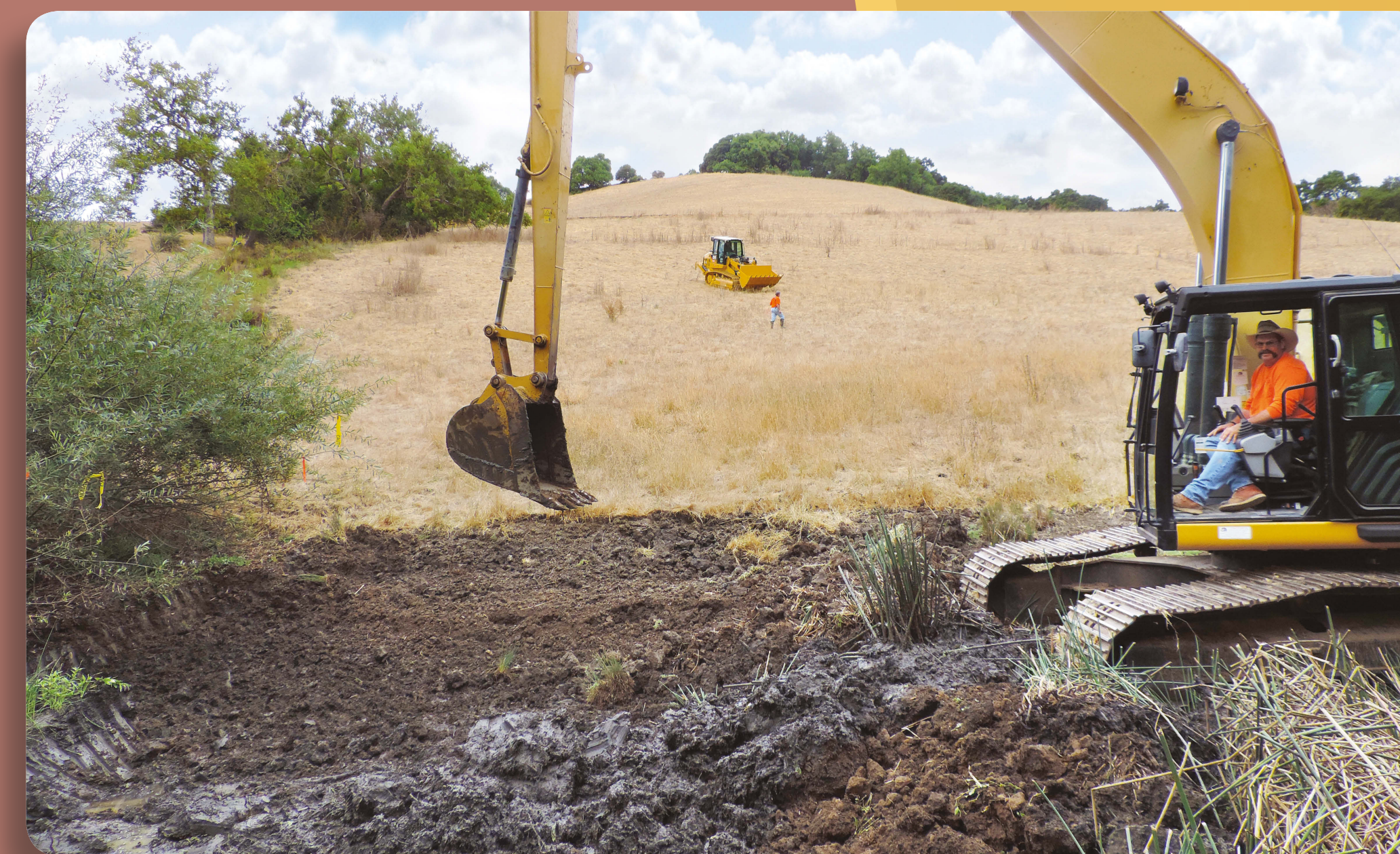
Figure 2. Pond restoration efforts using an excavator and Loader. Photo: D. Riensche
