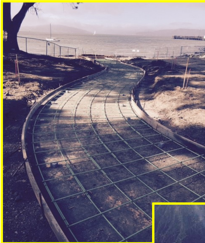
Second phase of regrading the path.
