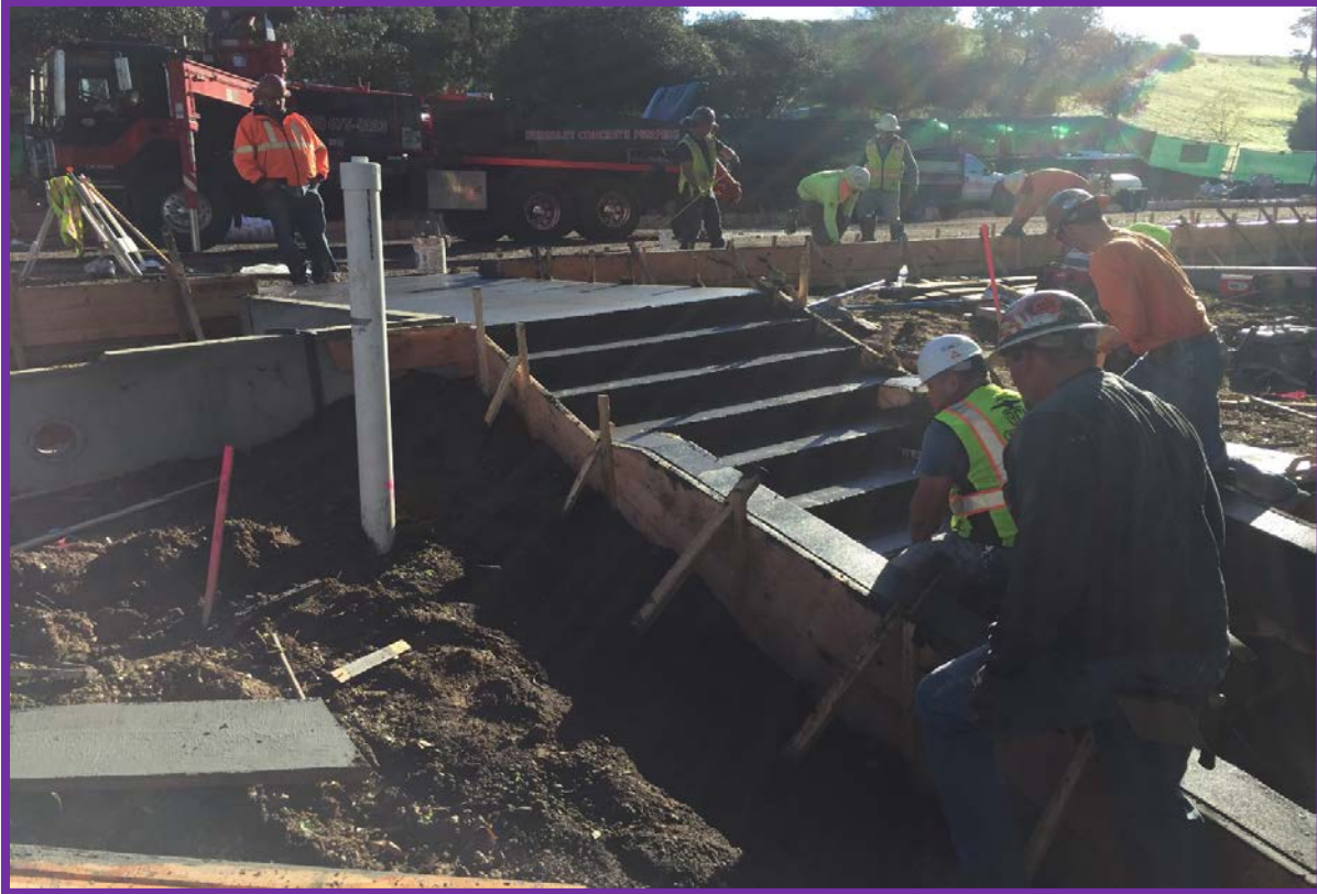
Constructing the stairs from the sidewalk to the building.
