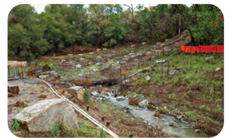
Plants sprout along the newly daylighted creek.
